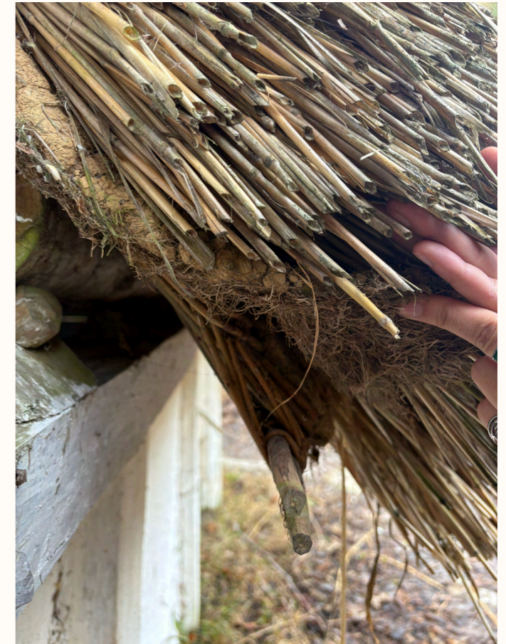
Layering of thatch and reeds on a roof
