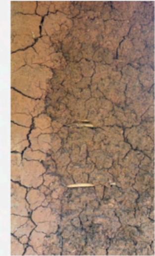
Mud on Reed Structure Wall, Ugandan Form of Bajareque
