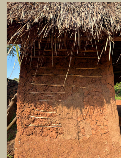
Textural details of the daub surface. (rough, smooth).
