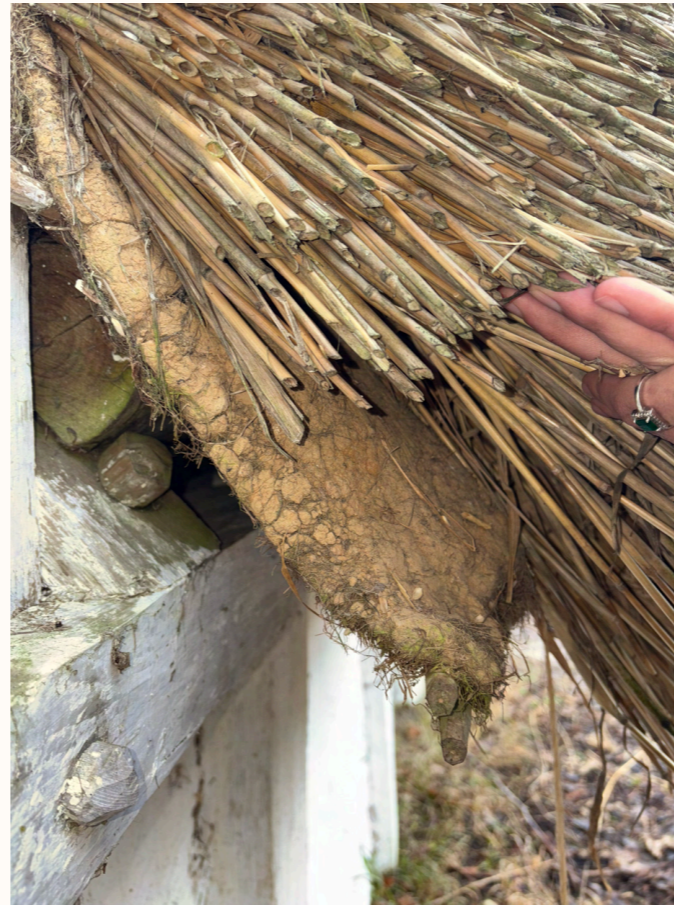
Layering of thatch and reeds on a roof
