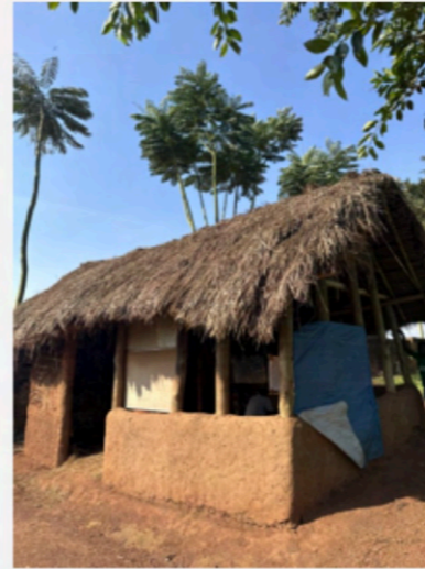
Traditional Hut Building Made from Natural Materials Of Thatch, Reed, and Mud
