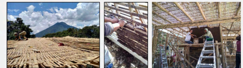
Bamboo School Project - San Pablo La Laguna, Guatemala
